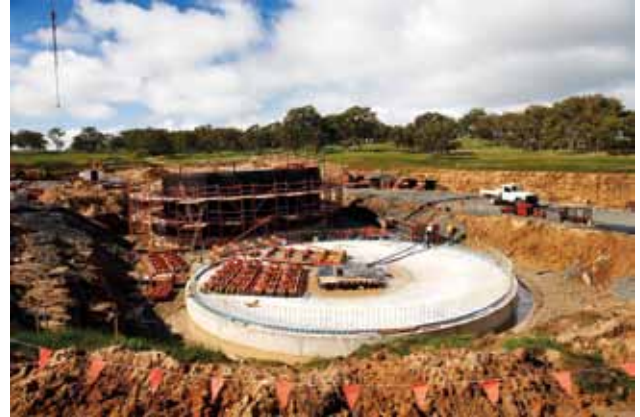
Clarifiers A and B.
