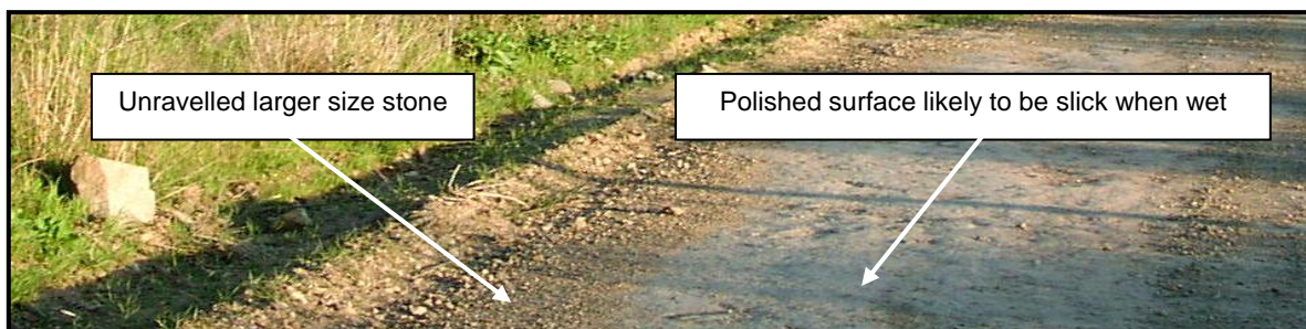
Figure 3.1 - Illustration of Quarry Waste used as Road Surface.
