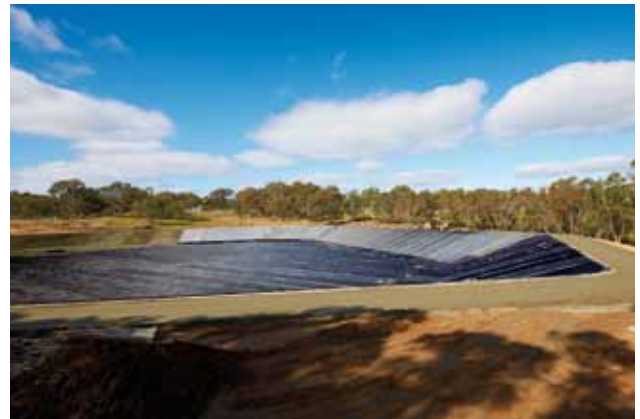
Reused water storage lining completed
