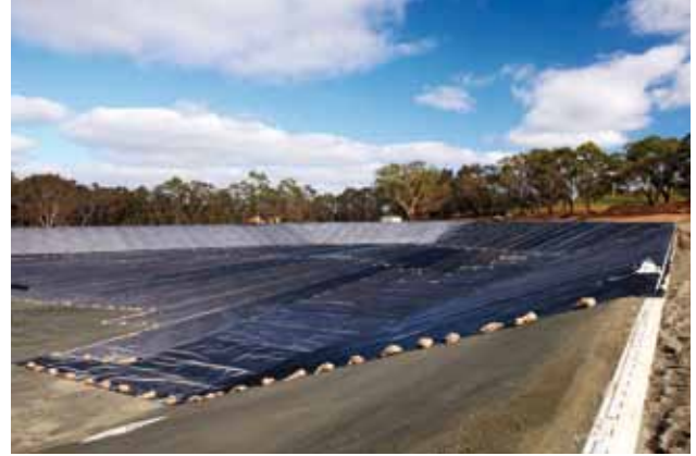
Reuse water storage lining
