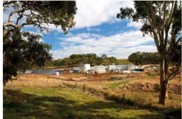
Treatment plant viewed from the west
