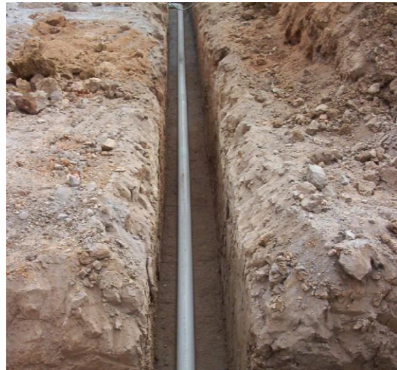
Example of Properly Bedded Drain
