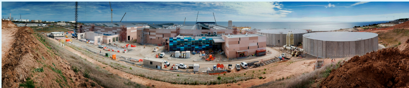
Adelaide Desalination Plant construction site
