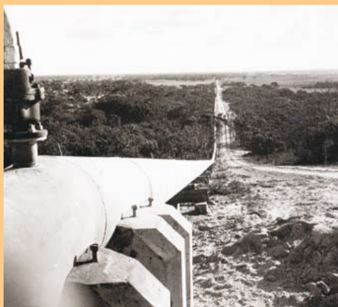
Above - Taillem Bend-Keith Pipeline. 21" MSCL pipe, looking West from near Sugarloaf Hill. July 1969.
