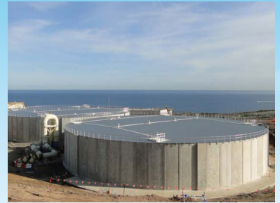
Water storage tanks
