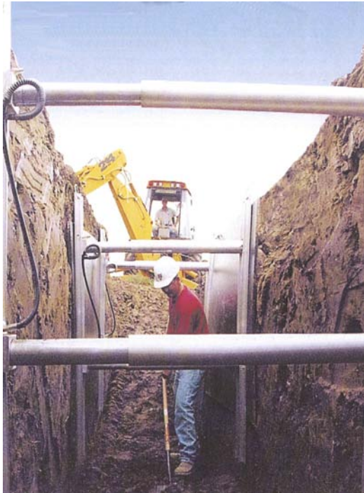
Figure 4.4 Metal Open Sheetting (Vertical Shores)
