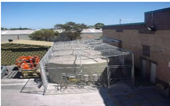
Aerial view of the storage tanks
