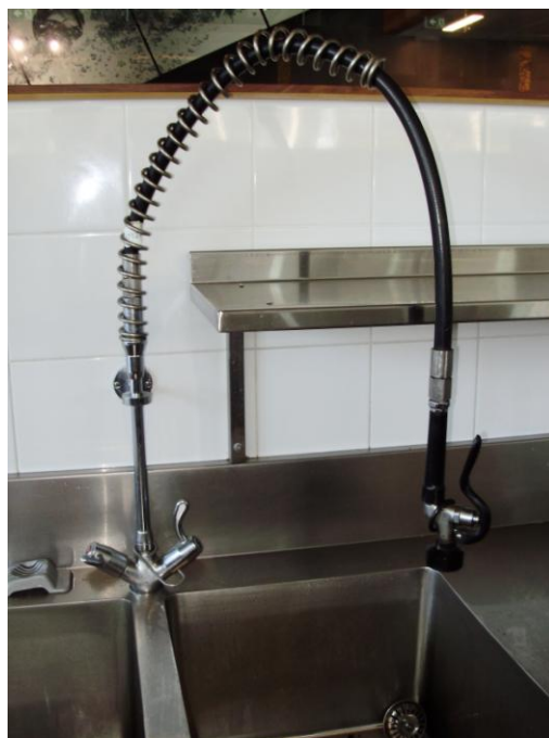
6 Star WELS rated pre-rinse spray gun (4.5L/min)
