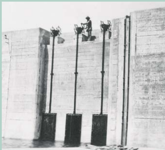
Above - Lock No. 1 Blanchetown. Valves, downstream end of Lock. December 1919.
