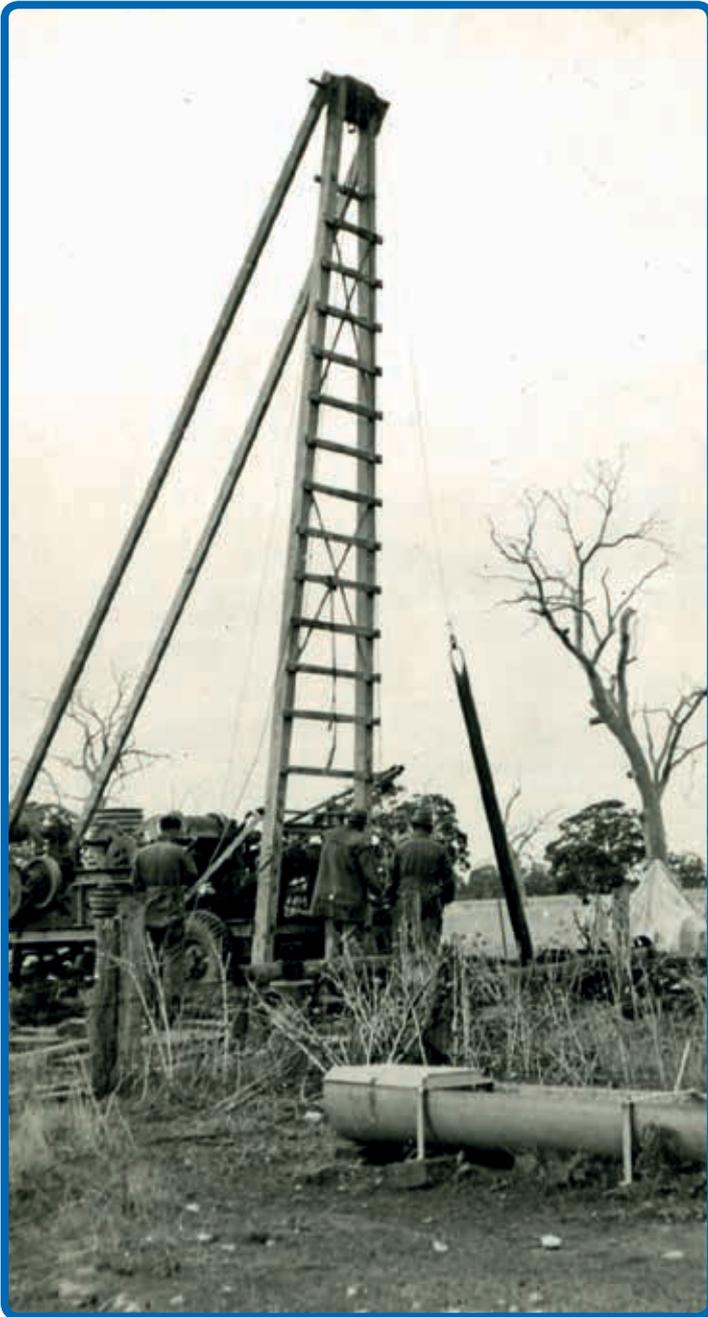
Construction of an 8 inch water supply bore.
