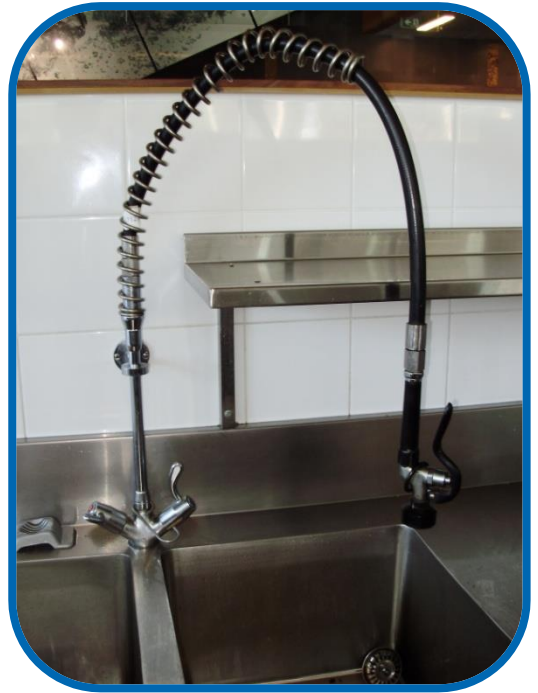
6 Star WELS rated pre-rinse spray gun (4.5L/min)
