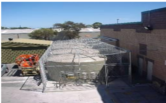
Aerial view of the storage tanks
