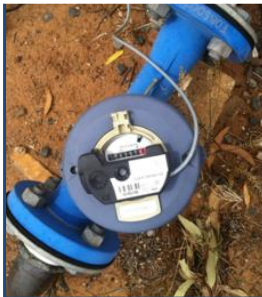
Figure 1: Data logging sensor on a meter
