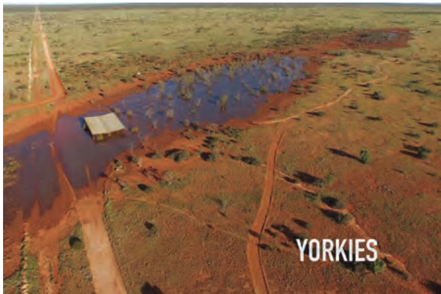
Aerial view showing former water storage 'shed tank'. Three bores located in the water to the left of the shed structure.
