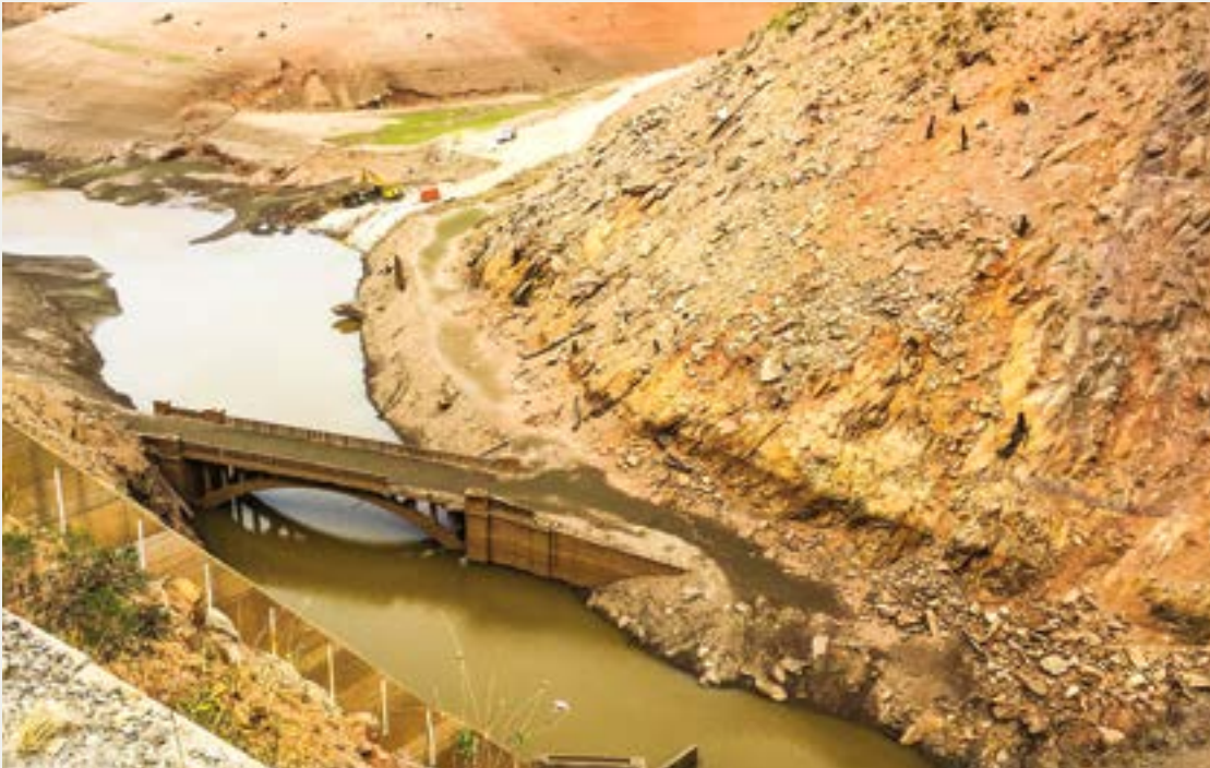
Bachelor's Bridge was exposed during works on the Kangaroo Creek dam upgrade.
