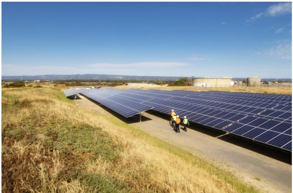
find solar panels attached to a mounting structure, connected to a row of piles in the ground. This may look a bit different depending on the technology being used.
