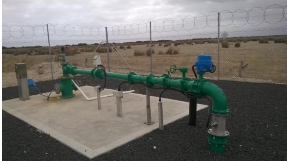
Figure 5: Typical view of a headworks and concrete slab / plinth
