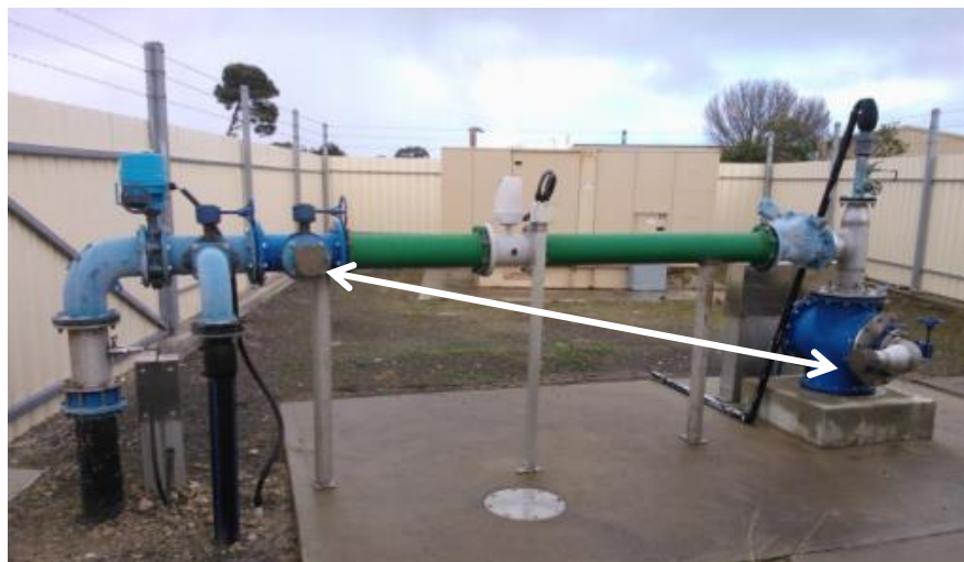
Figure 7: Provision of headworks recirculation loop
