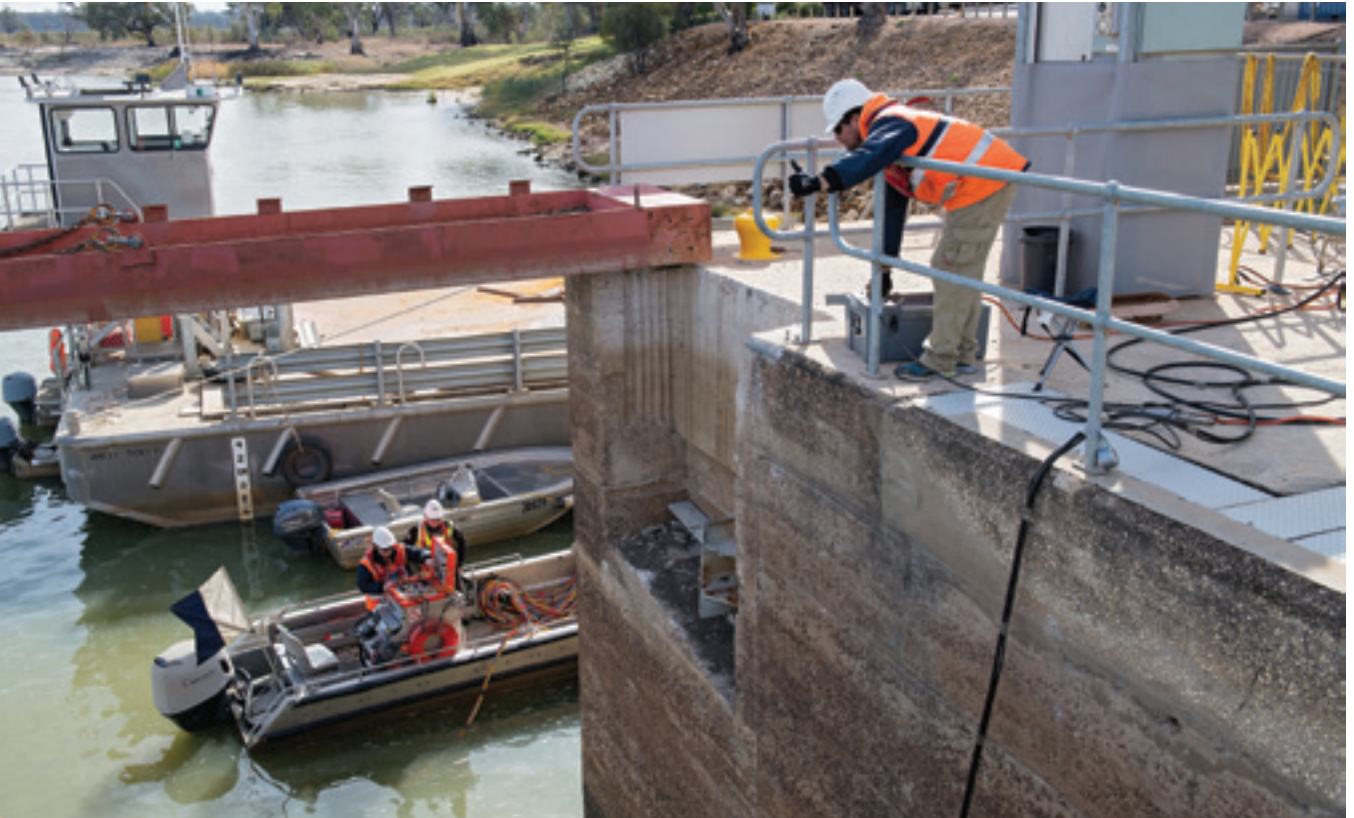
The refurbishment of Lock 3.
