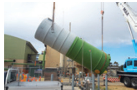
Below: The new trickle filter is lifted into place at the Port Adelaide Wastewater Pump Station.
