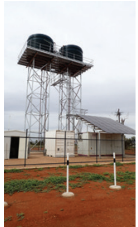
The new water storage tanks in Watinuma.
