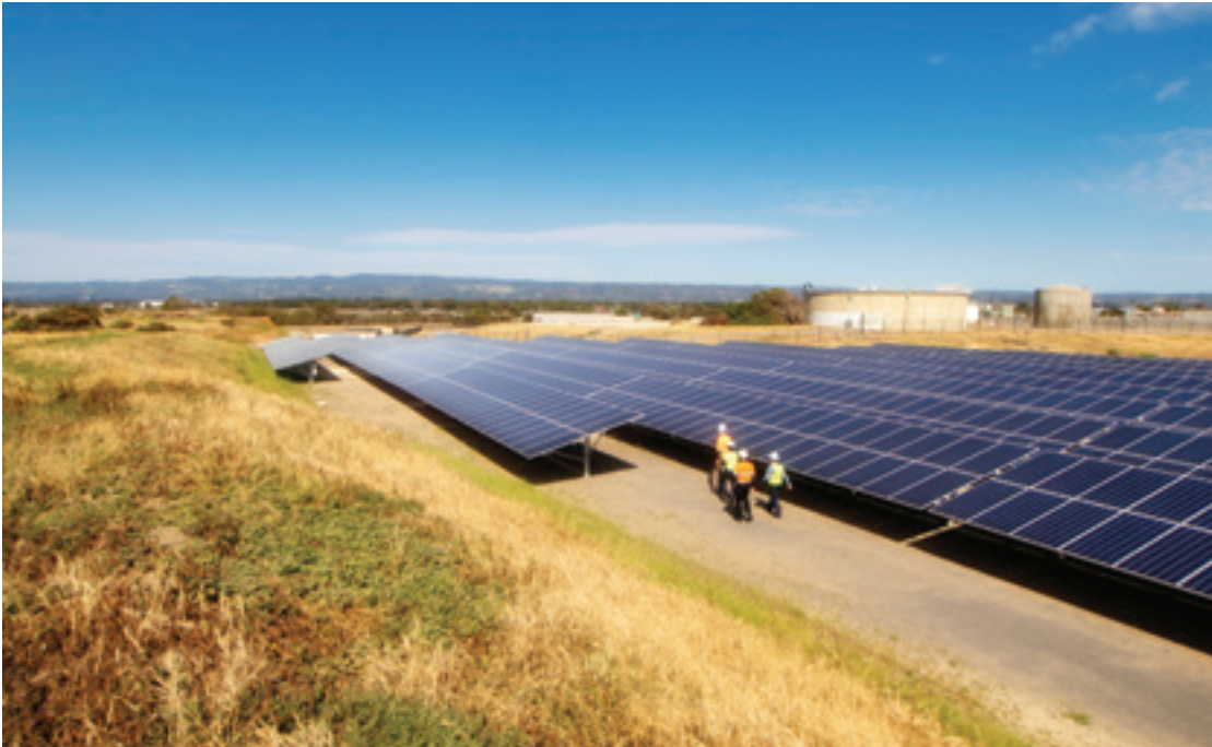
Left: The solar array at Glenelg Wastewater Treatment Plant.
