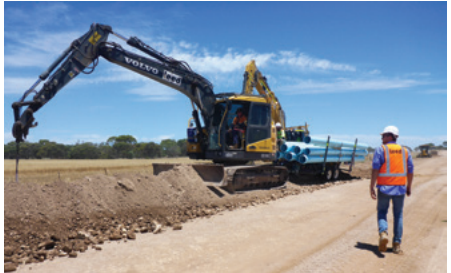
Warooka pipeline construction on Hardwicke Bay Road.
