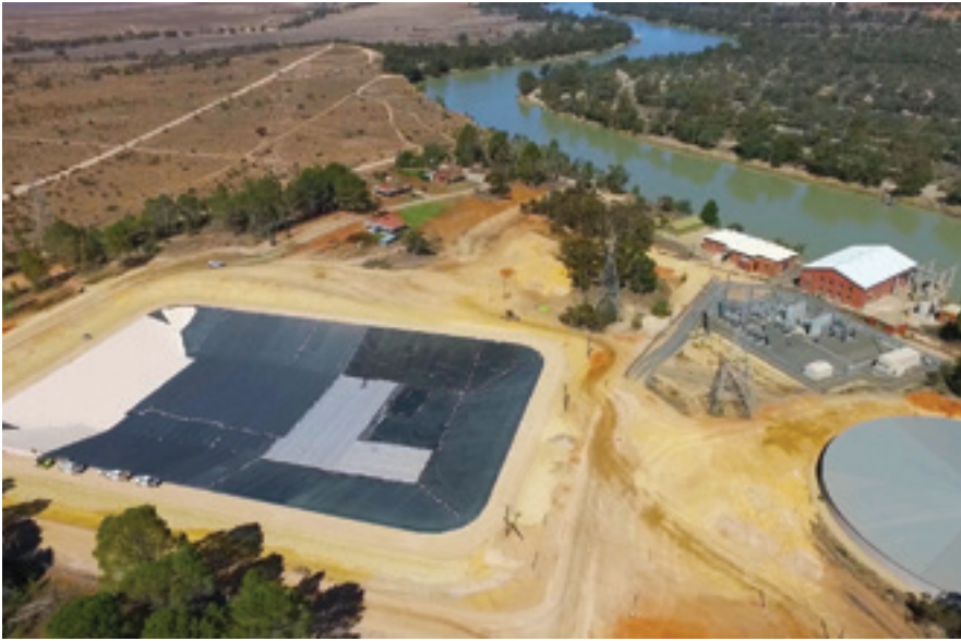
Above: The new earth bank storage at Morgan Water Treatment Plant.
