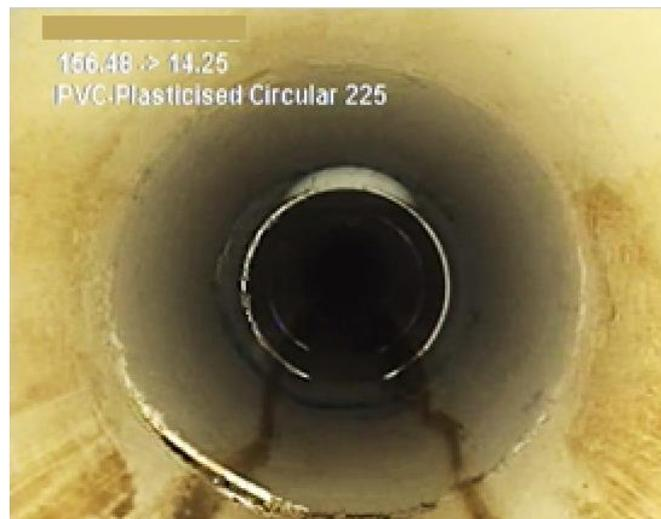
**Figure 10 Defective Joint Seal**
