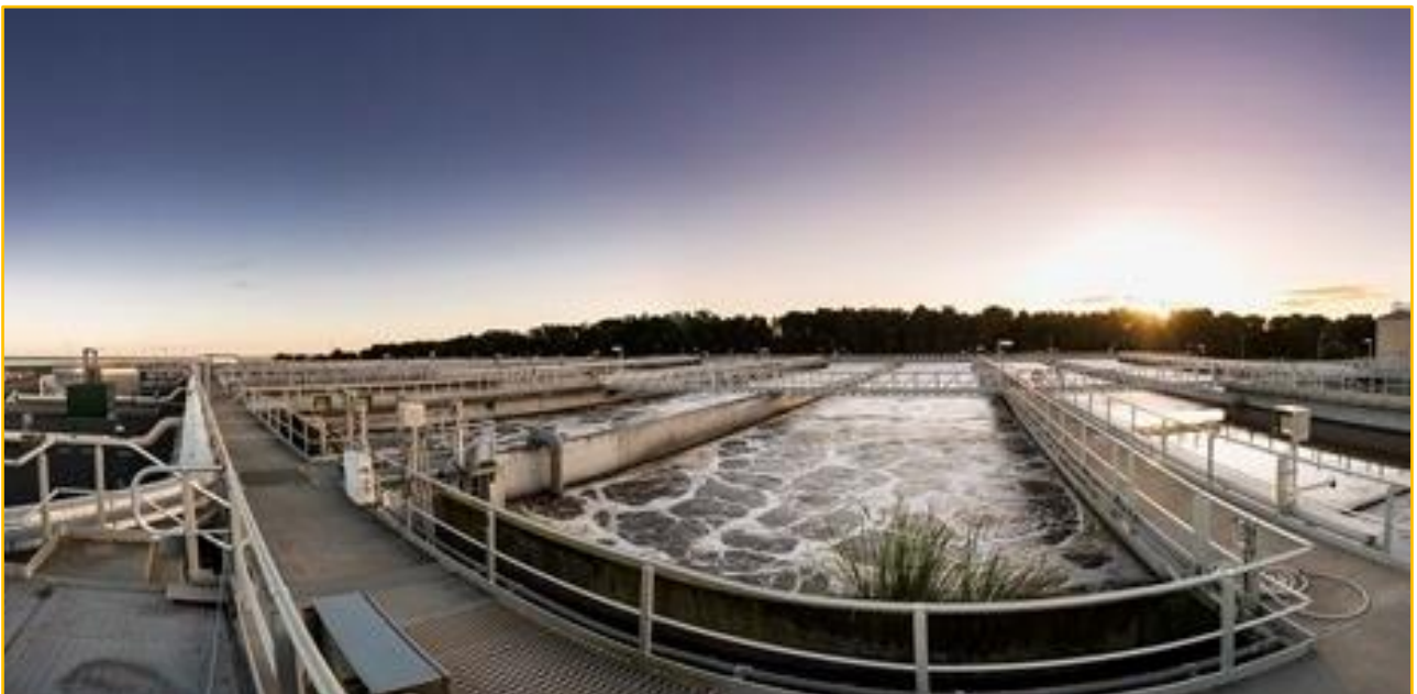
Aeration tanks operating in the wastewater treatment process
