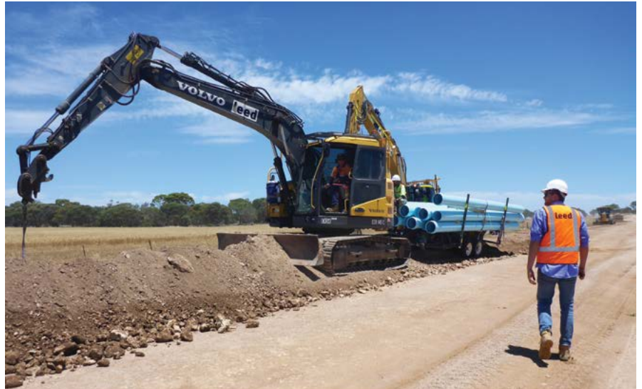
Warooka pipeline construction on Hardwicke Bay Road.
