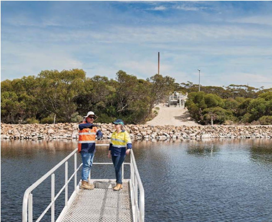
Left: Construction is underway on the final stages of the Port Lincoln Wastewater Treatment Plant upgrade.
