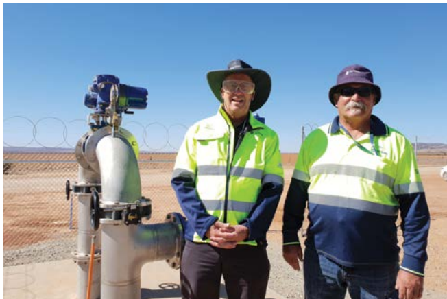
Right: General Manager Asset, Operations and Delivery Mark Gobbie and District Leader for Clare and Mid Murray David Daly with new Orroroo pipeline infrastructure.
