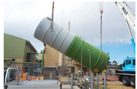
Below: The new trickle filter is lifted into place at the Port Adelaide Wastewater Pump Station.
