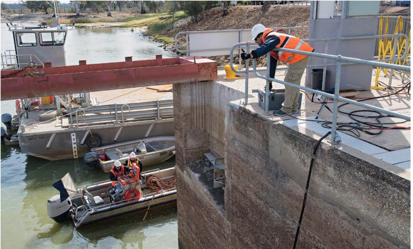
The refurbishment of Lock 3.
