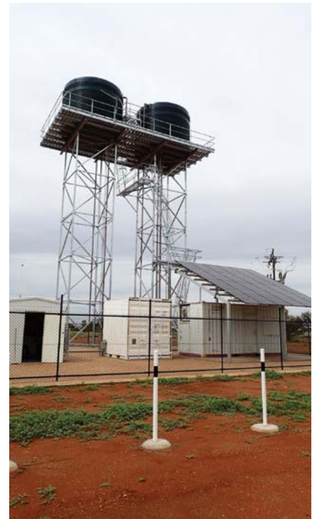
The new water storage tanks in Watinuma.
