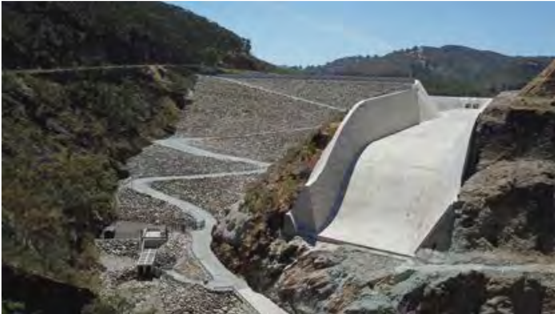
The new spillway at Kangaroo Creek Dam.
