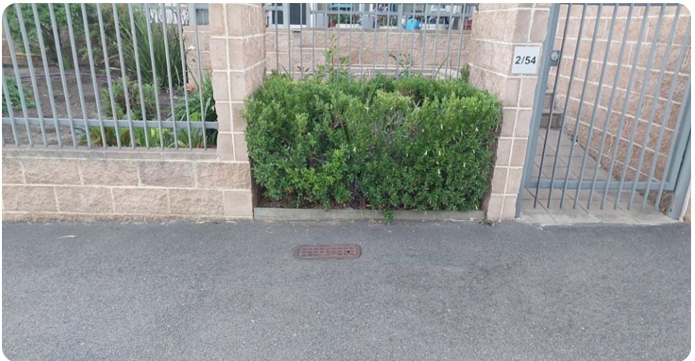
Example of water meter in box
