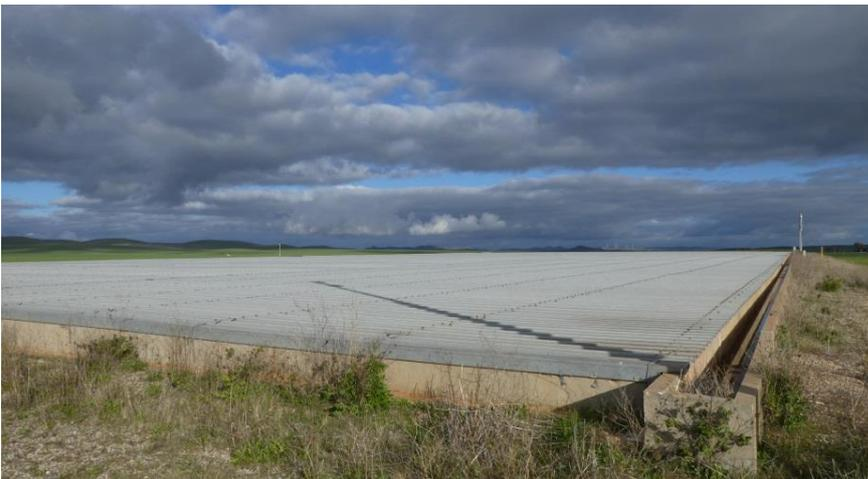
**Figure 8: EBS with concrete liner and fixed roof (Hanson)**
