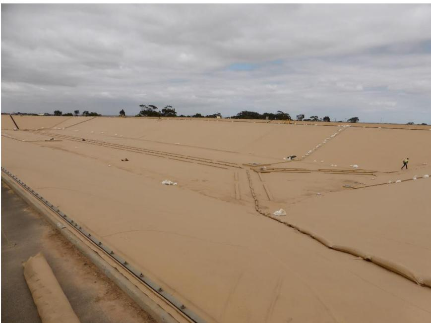
**Figure 4: Geomembrane lined and covered storage (Upper Paskeville)**
