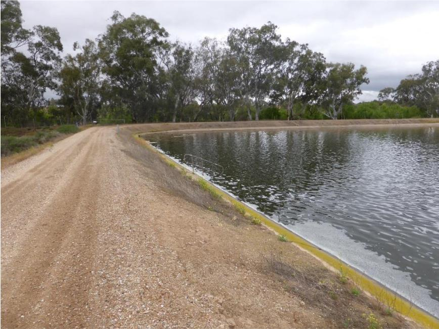
**Figure 7: EBS with concrete liner (Mannum WWTP)**
