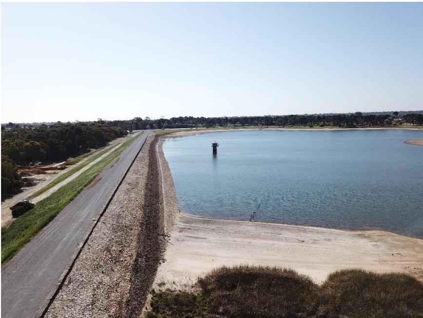
**Figure 1: Hope Valley Dam, zoned earthfill dam with puddle clay core**
