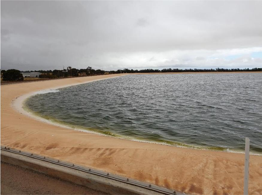
**Figure 5: Geomembrane lined storage with no cover (NAIS)**
