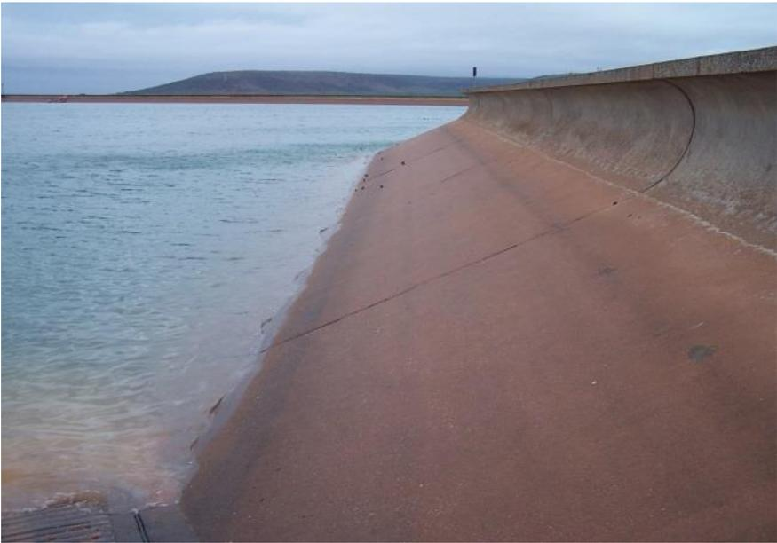
**Figure 6: EBS with concrete liner (Lincoln Gap)**
