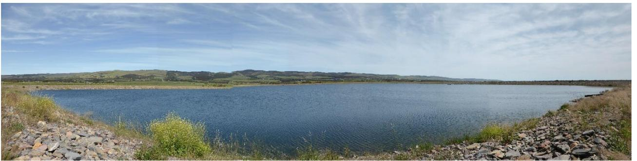
**Figure 3: Earth embankment with riprap protection (Aldinga WWT, Lagoon 3)**
