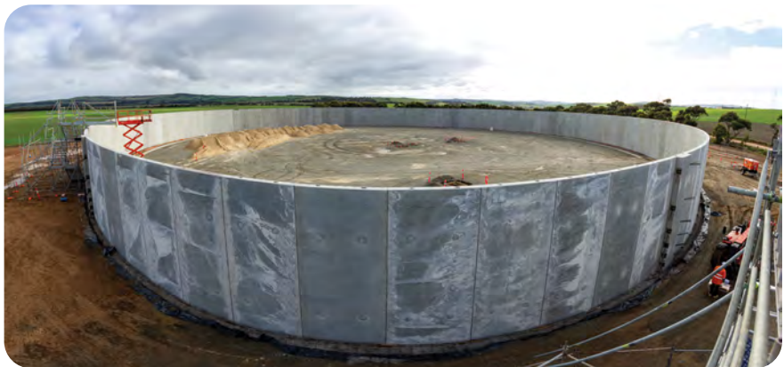
The Green Patch tank's 112 concrete panels were craned into place.
