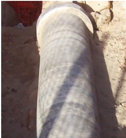
Photo 1: Asbestos cement pipe
