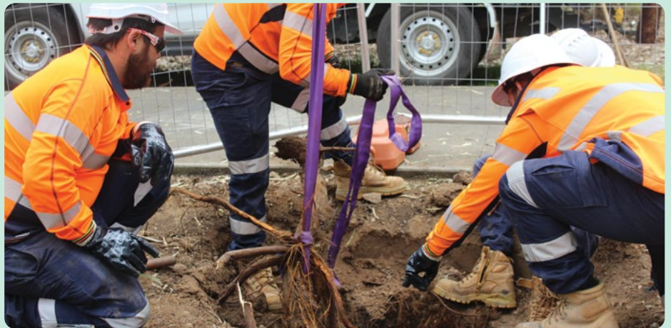
Tree roots remain the leading cause of sewer blockages across our wastewater network.
