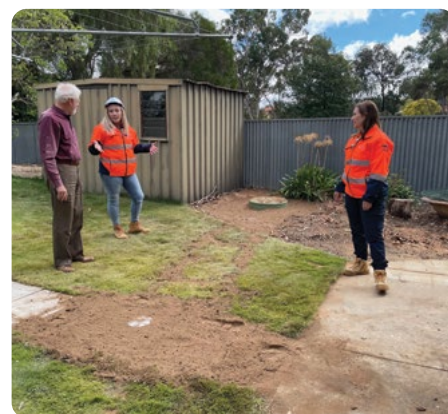
New sewer connections are helping improve wastewater services for Tea Tree Gully communities.
