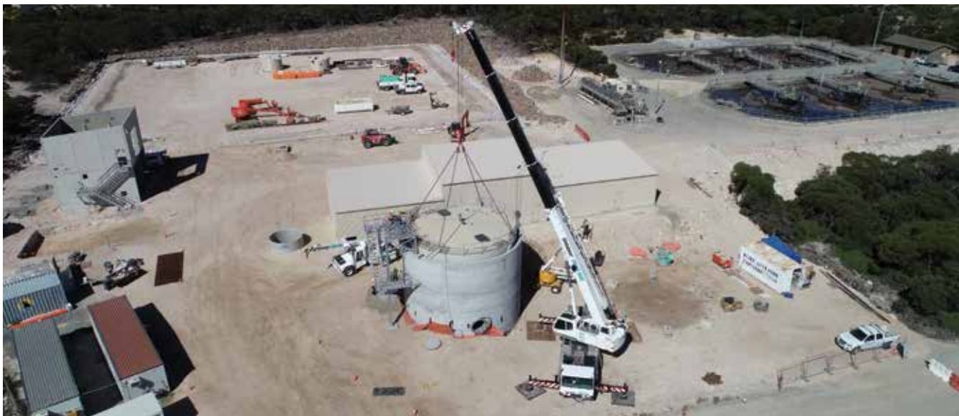
The anaerobic digester's 20 tonne steel cover was carefully guided into place with the help of a locally-sourced mobile slew crane.
