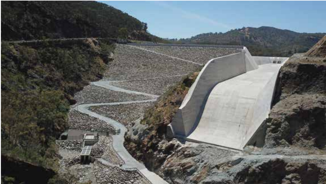
The new spillway at Kangaroo Creek Dam.
