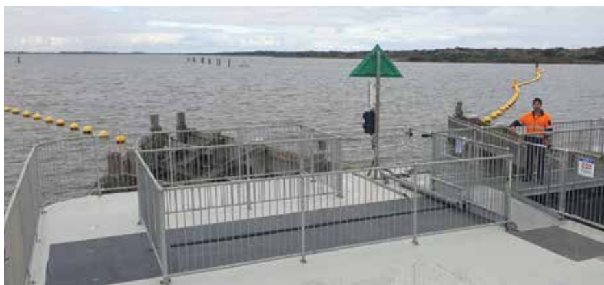
The new access platform at the Goolwa Barrage enables visitors to safely walk on both sides of the barrage.
