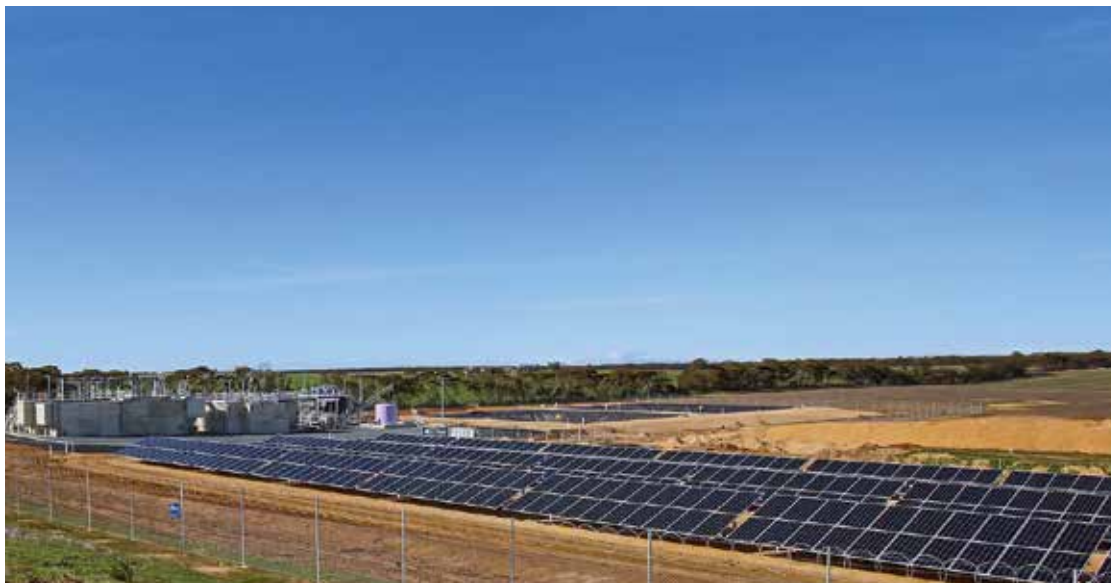
Left: The new Murray Bridge Wastewater Treatment Plant is a leader in sustainability design.
