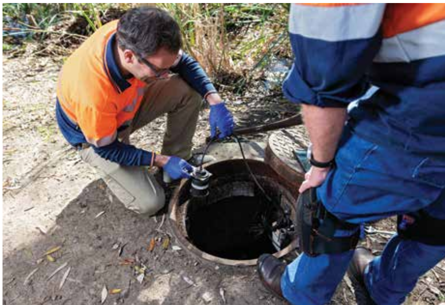
Left: Sensors installed in the wastewater network are helping reduce customer impacts from sewer blockages.
