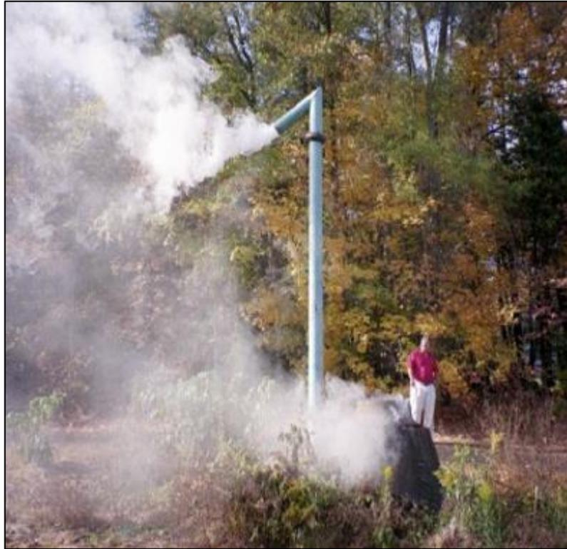
**Figure 7-4 Uncontrolled Air Release Caused by Hydraulic Surge**
