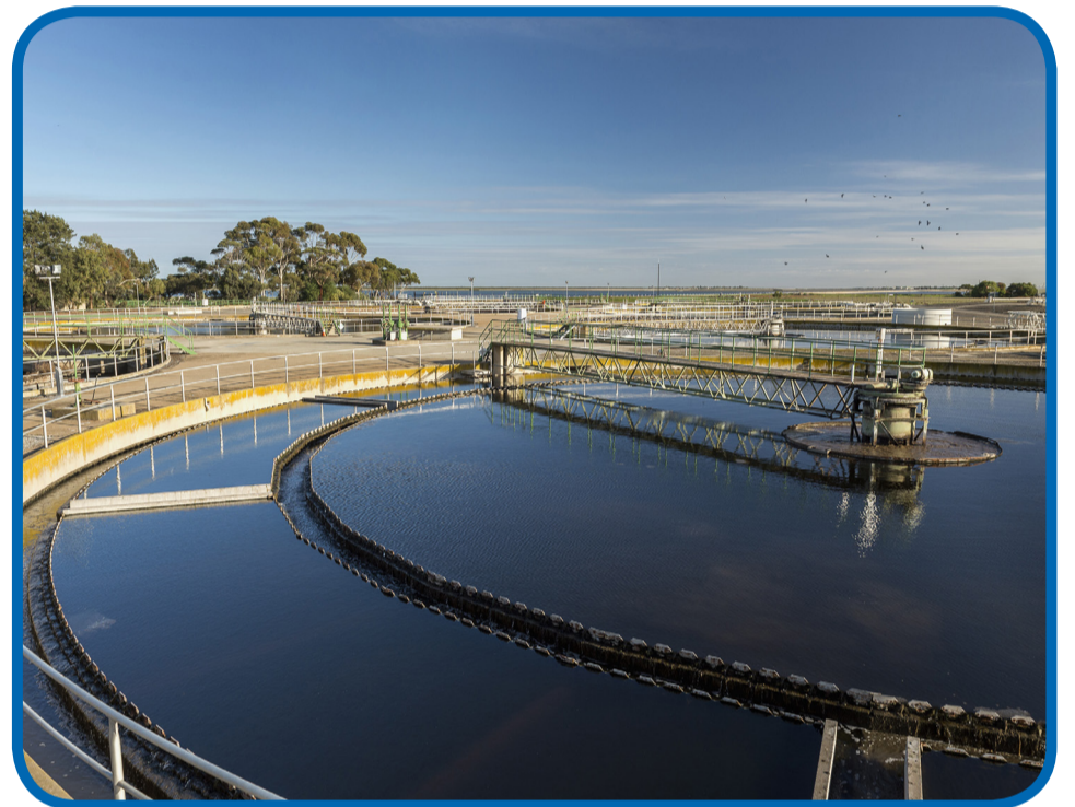
Wastewater is passed through the above clarifiers during the secondary treatment process at the Bolivar Wastewater Treatment Plant
