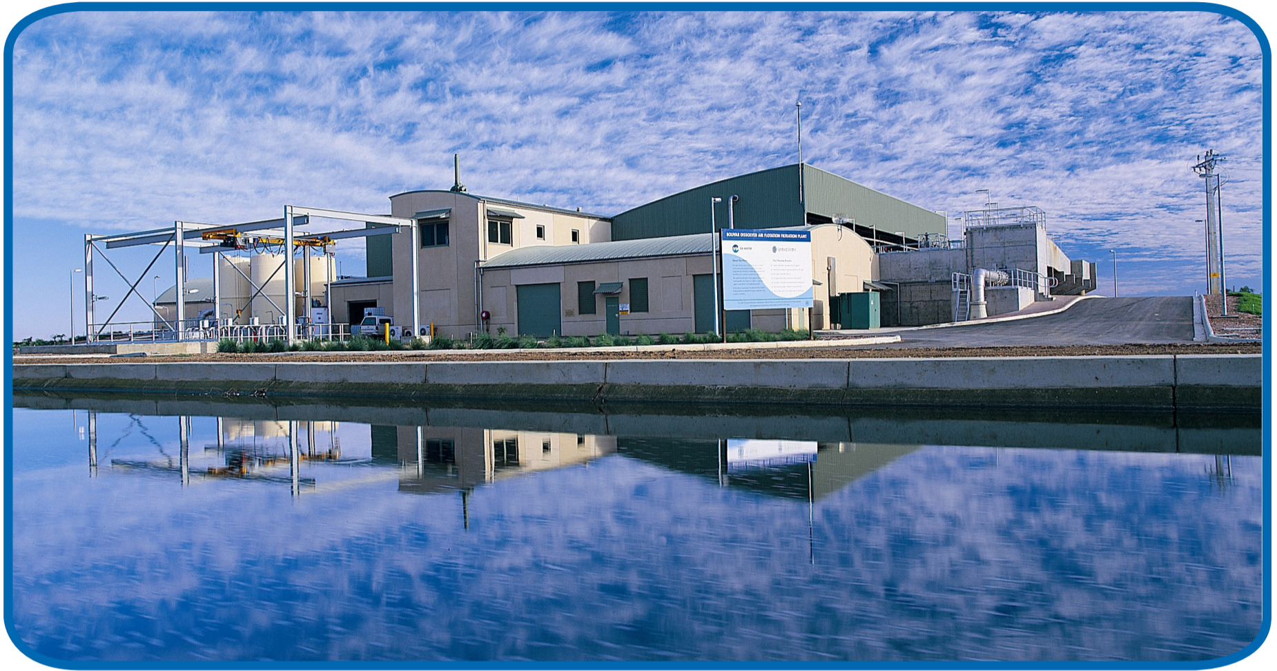
Additional winter water can be made available to the NAP community from the existing Dissolved Air Floatation Filtration (DAFF) plant at Bolivar.
