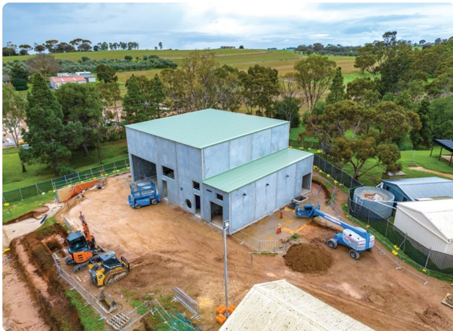
Major upgrades at Gawler East are strengthening water services for future growth.
