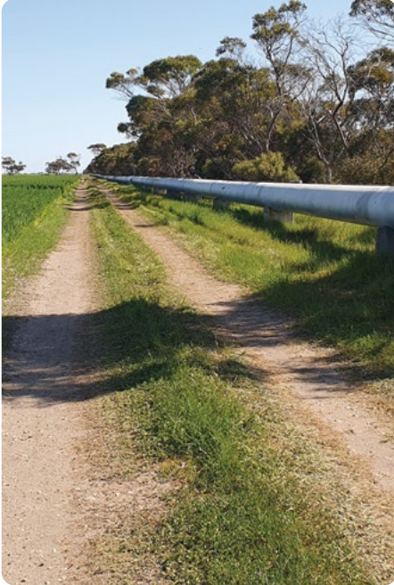
The completed Tailem Bend to Keith Pipeline upgrade will improve water reliability for regional communities.
