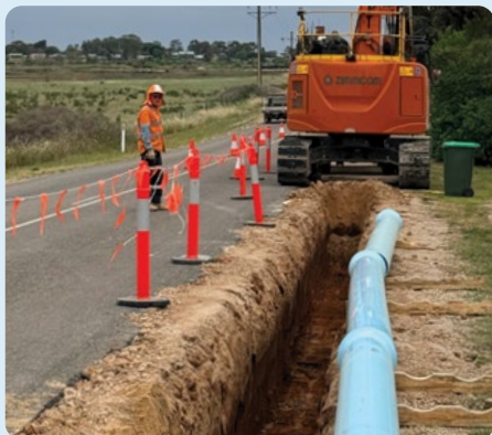
New water infrastructure has connected Wellington East to our drinking water network.
