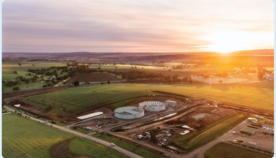
New water storage at Sandy Creek will help meet growing demand across northern Adelaide and surrounding communities.
