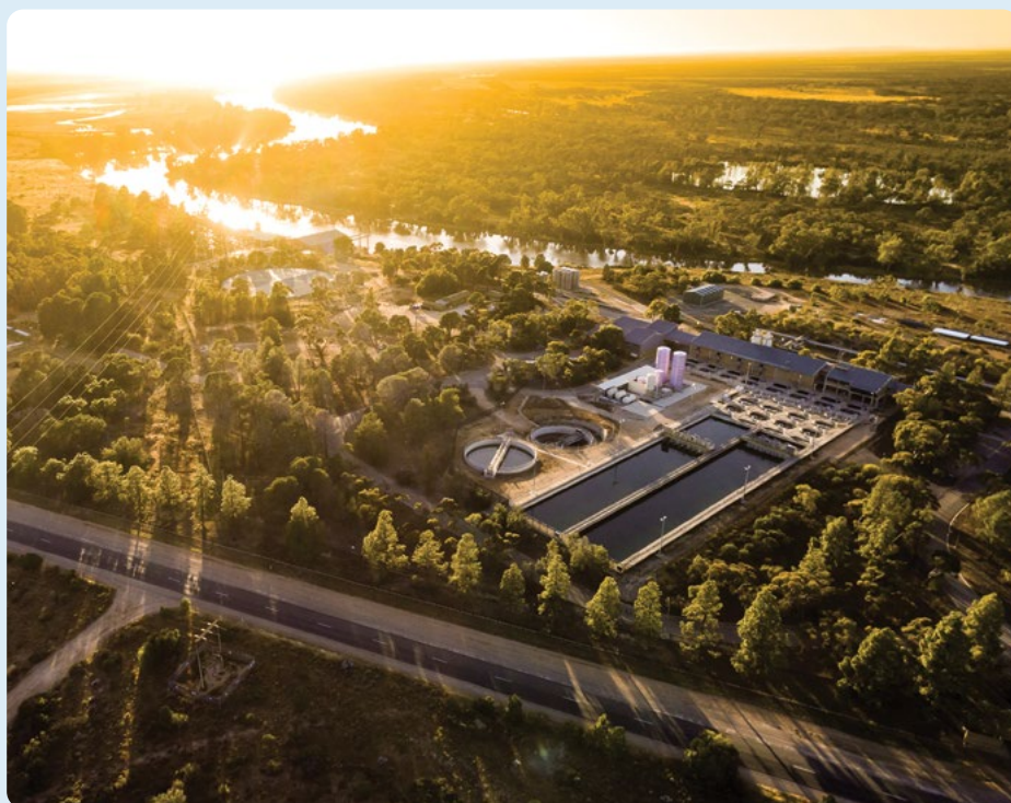
Morgan Water Treatment Plant produces approximately 40 per cent of the drinking water supplied across regional South Australia.
