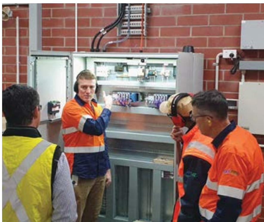
The onsite condition-based monitoring control panel at Murray Bridge which houses equipment that collects data from sensors on pump sets.
