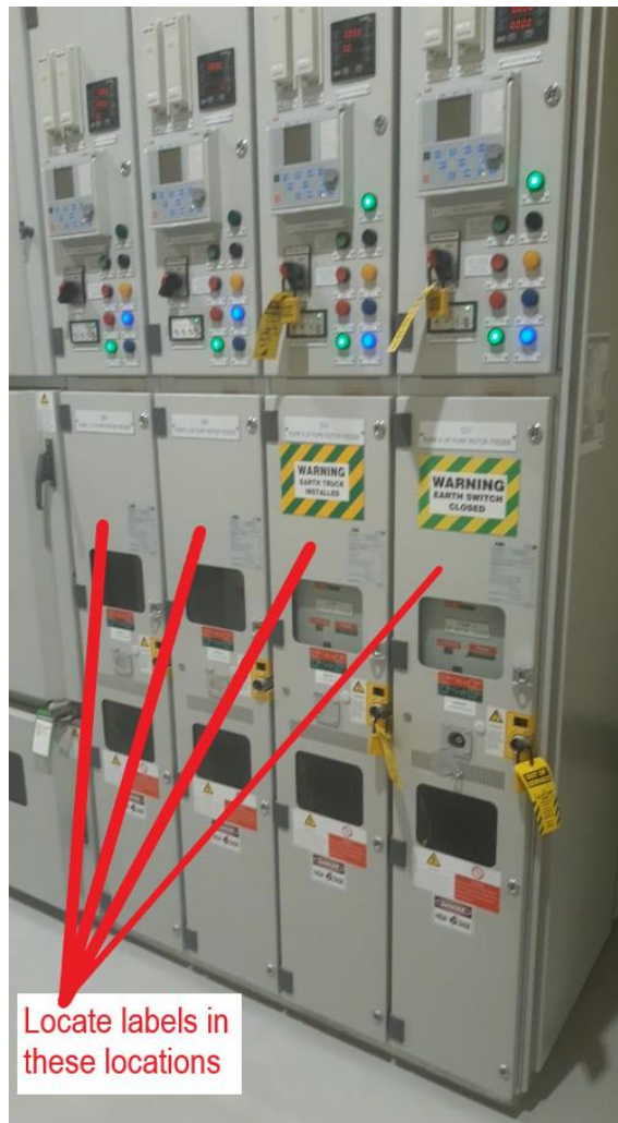
Figure 6-7: Example positioning of warning labels
