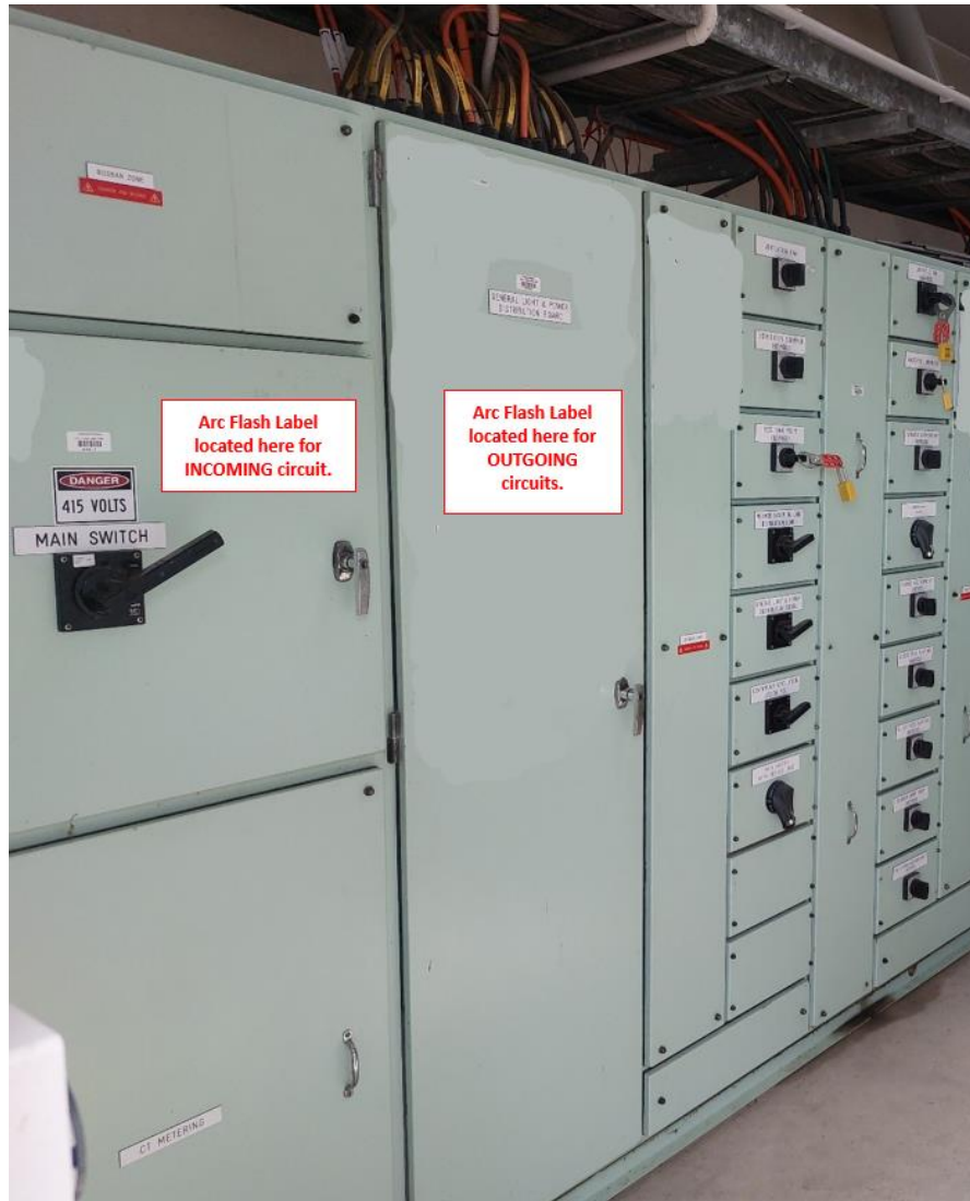
Figure 6-3: Example positioning of arc flash labels
