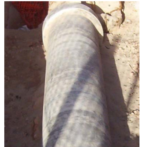
Photo 1: Asbestos cement pipe
