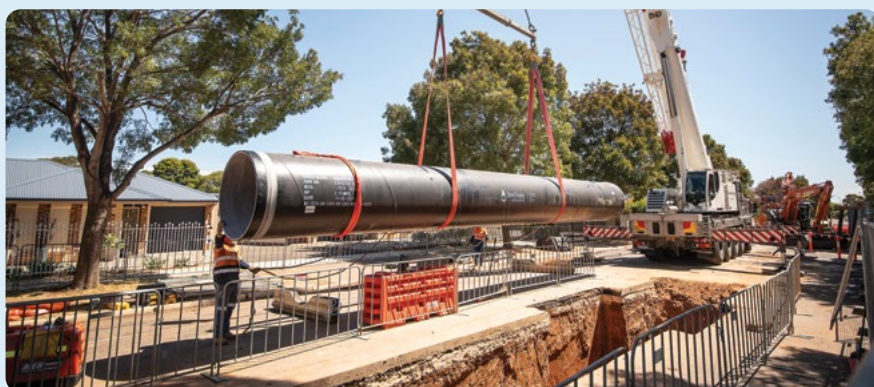
Pipe installation underway to support a major network expansion that will enable new housing across Adelaide's northern suburbs.
