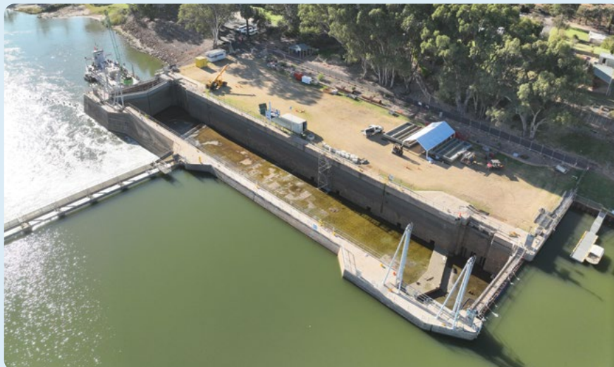
Lock 3 has been dewatered to enable maintenance on the 100-year-old asset.
